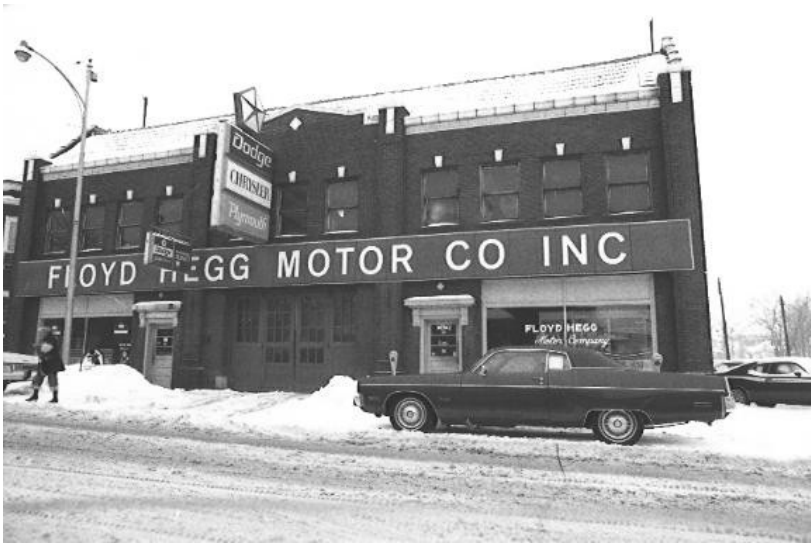
225 N. Central *, with car lot on north side
