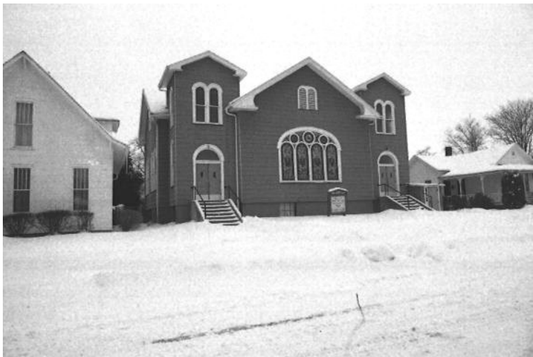
Otterbein Methodist Church on Washington St, houses on either side are gone
